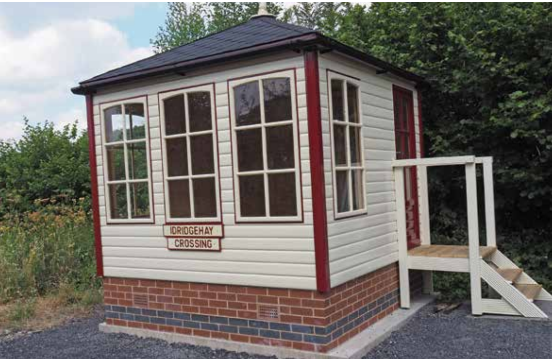
New Crossing Keeper Box at Idridgehay.
