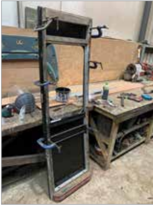
Door metal and wooden frames re-united.
