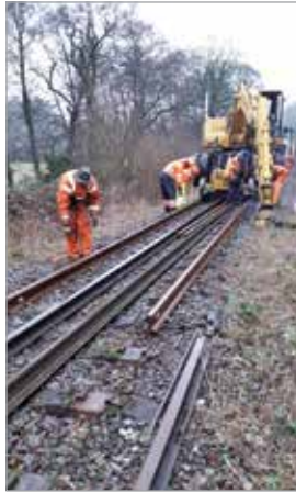
All above: Fitting and cutting test rails.
