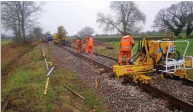
The P-Way team in action with the rejuvenated slewing machine.
