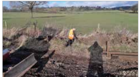
Hand excavation for drainage
