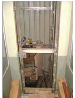
Door inner frame after timber repair
