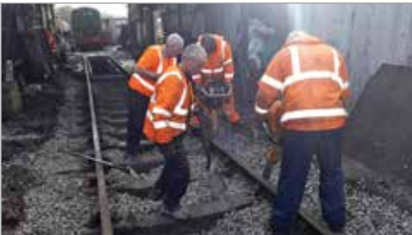
Hand ballasting at the shed
