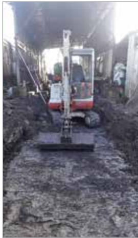
Removal of slurry and levelling at steam shed.
